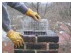
The HSUS Installing a chimney cap.
